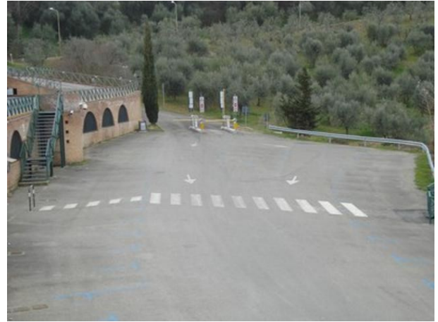
Parking P4 Bagnaia inferiore
